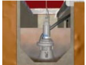
*Pump with internal cooling system*
