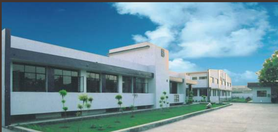
Roto's Manufacturing Plant
