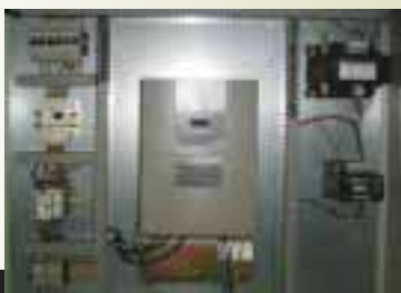
4 level control built into a control box
