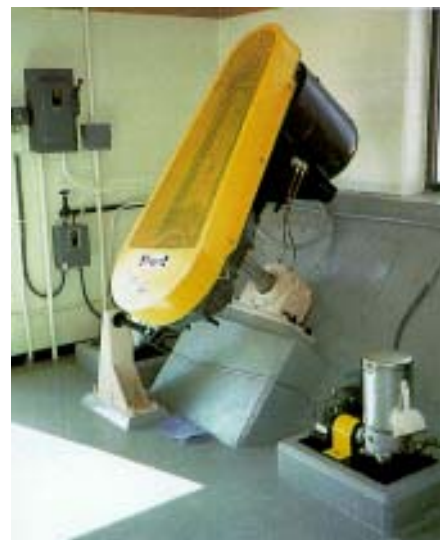
Lakeside's V-belts act as a shock absorber in the drive system.
