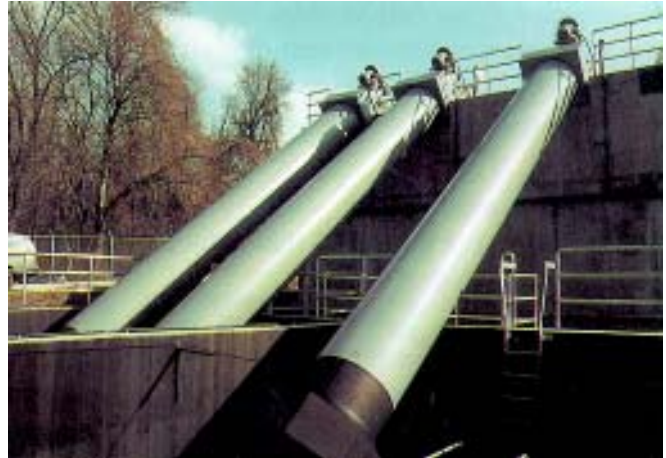
Enclosed screw pumps are capable of operating at 45° inclinations.
