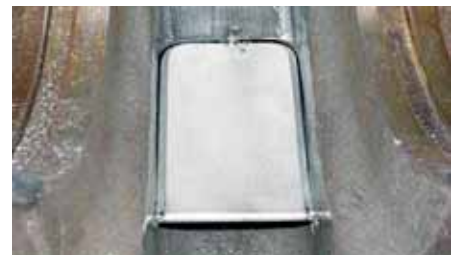
New volute lip extension tacked in place
