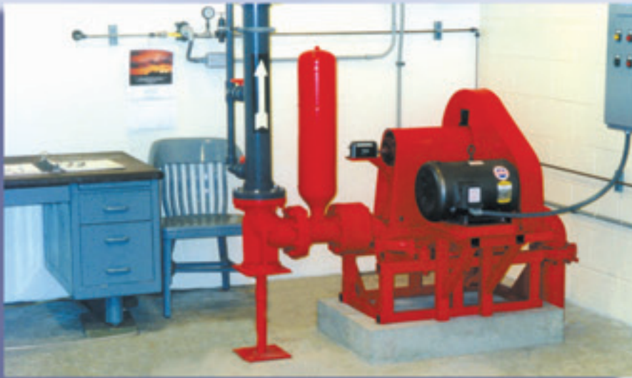
Town of Caernarvon, PA WWTP
